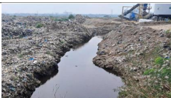
Figure 5. Unlined trenches pose a groundwater risk at the Perungudi dumpsite [40]
