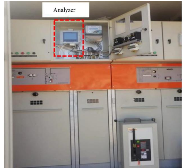
Figure 4. Installation of data collecting unit.
