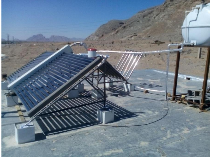
Fig. 1. Photo of the proposed desalination unit
