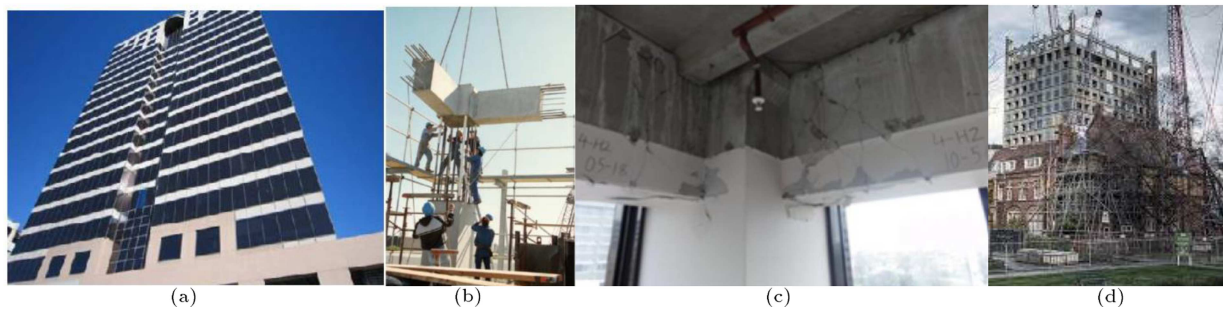
Figure 13. Precast emulative tower [62]: (a) Exterior; (b) construction; (c) typical seismic damage; and (d) demolition.
