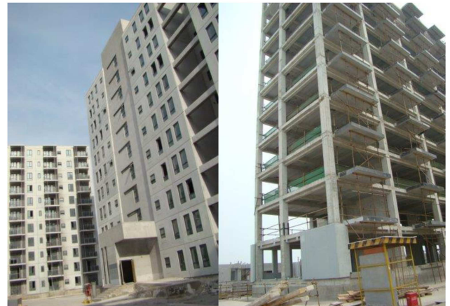
Figure 7. China precast projects [45].
