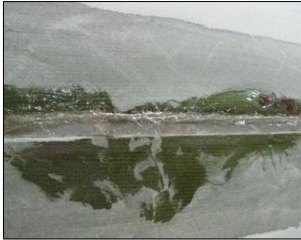
Figure 3 Application of roving in the repaired area
