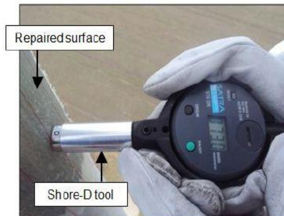
Figure 5 Final inspection of repaired leading edge to check for irregularities
