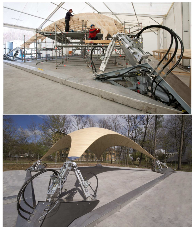
Figure 2. Adaptive thin shell structure with sensor and actuators under construction (top photo) and after completion (bottom photo) (Courtesy of Michael Heidingsfeld of Bosch Rexroth Company).
