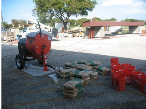
Figure 2. Site with equipment used for UHPFRC mixing in Miami (US)
