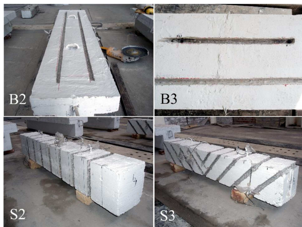
Figure 5. Cutting the groove of RC beams.
