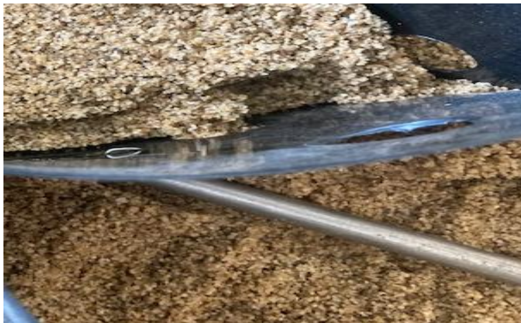
Fig. 5. Wire attachment to the geocell wall
