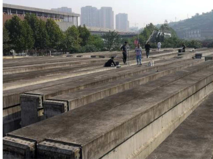
(b) The beam yard
