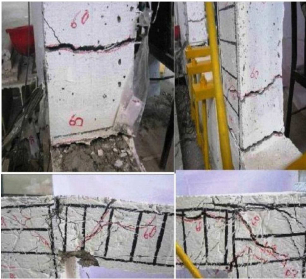
Figure 4. Location of cracks and tensile cracks pattern in experimental model [23].
