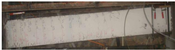
Fig. 3. Damage and crack pattern of specimens views
